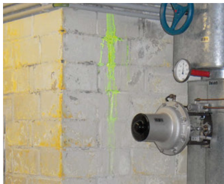
Detection of a leaky water-carrying pipe in a building by passing in uranine and performing a subsequent UV inspection.
