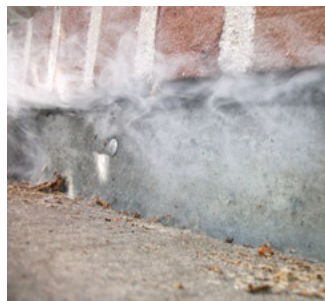
Evidence of defective sealing of the wall connection above an underground garage.
