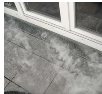
Defective sealing of a roof-top terrace.
